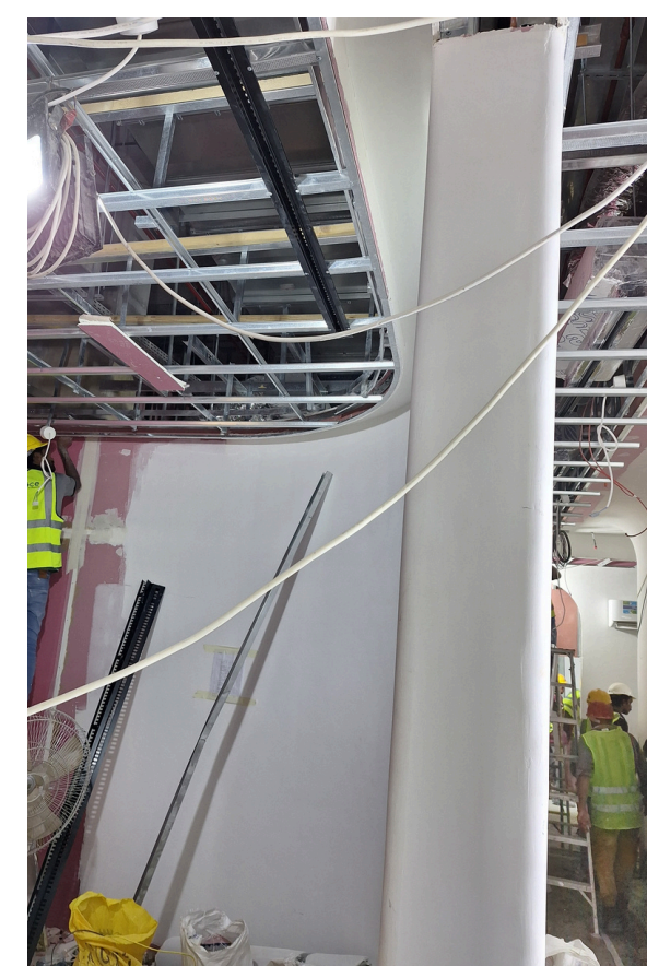
AVIDA LONGEVITY CLINIC JUMEIRAH- UNDER CONSTRUCTION
